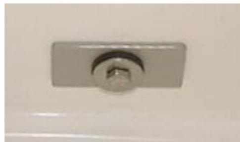
replacing the pin, place a ring of sealant around the pin on the inside surface of the aluminum only. The rubber washer will seal off any leak around the pin.
